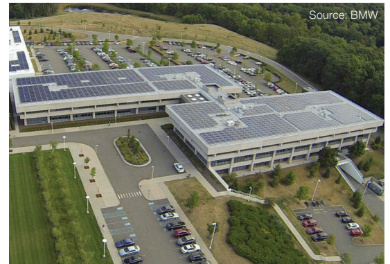
NextEra installed a 1.2-megawatt system on four rooftops at BMW's North America headquarters in Woodcliff Lake, New Jersey.
