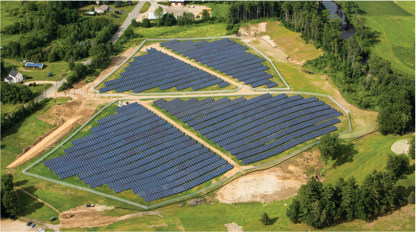
Hardwick Solar was installed on a private golf course in Massachusetts.
