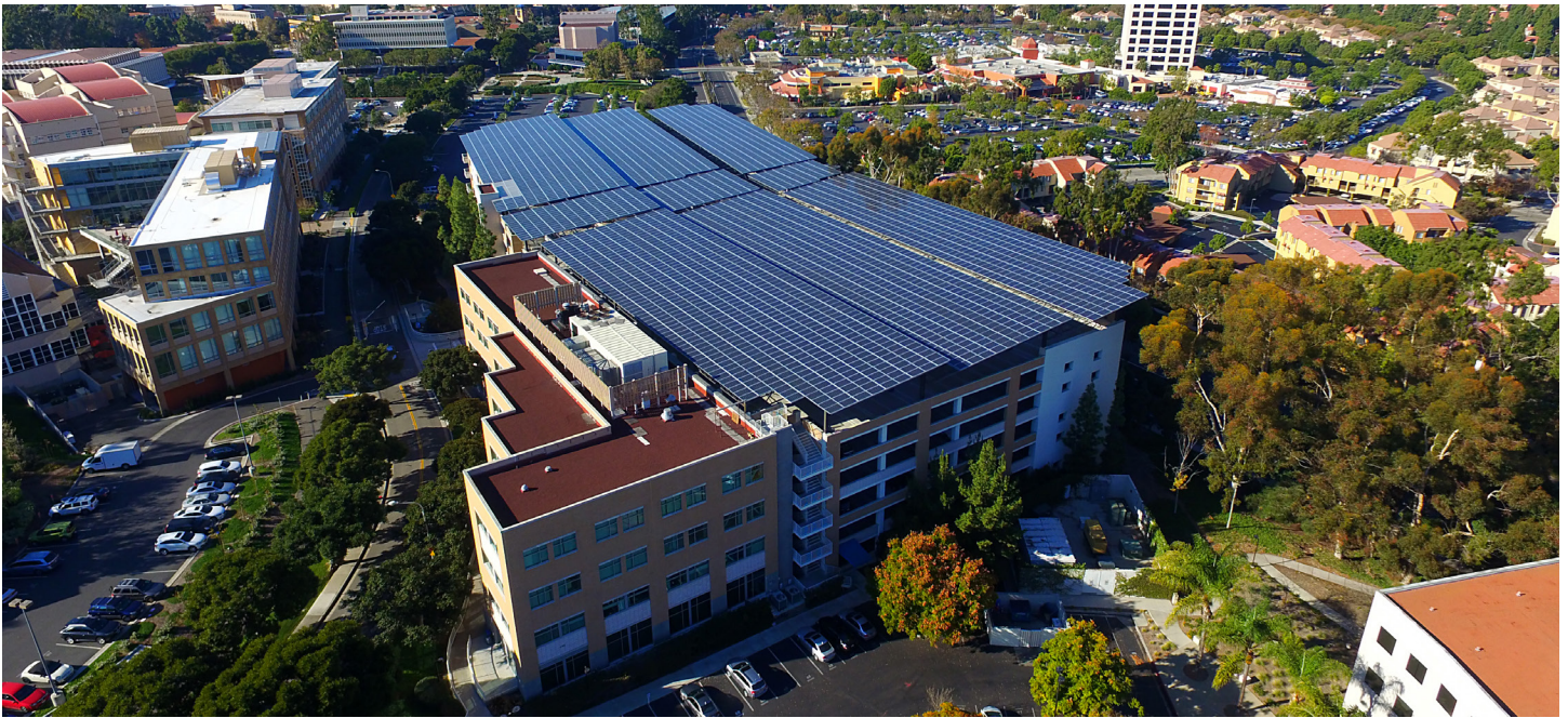
DG solar installations add value to available roof space.
